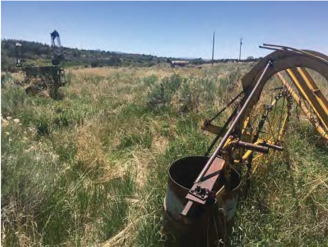
Description: Drainage AST and debris
