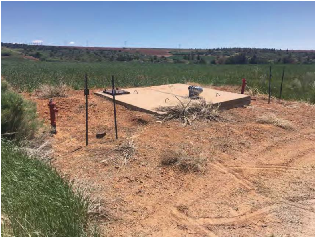
Description: Garcher underground structure
